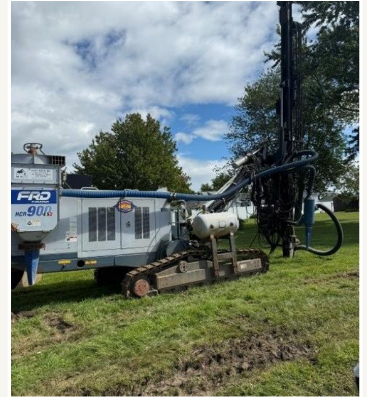
Directional drilling rig used to create the underground bore path.
